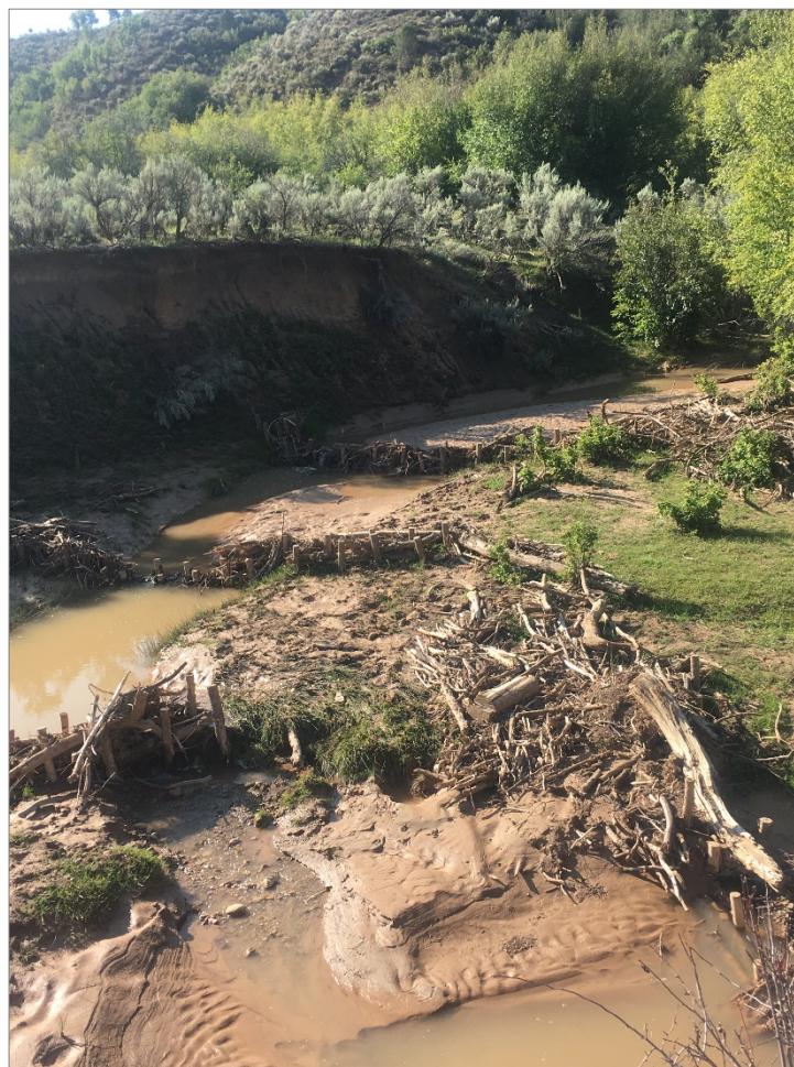
Beaver dam analogs (BDAs) hold sediment on Fish Creek.
