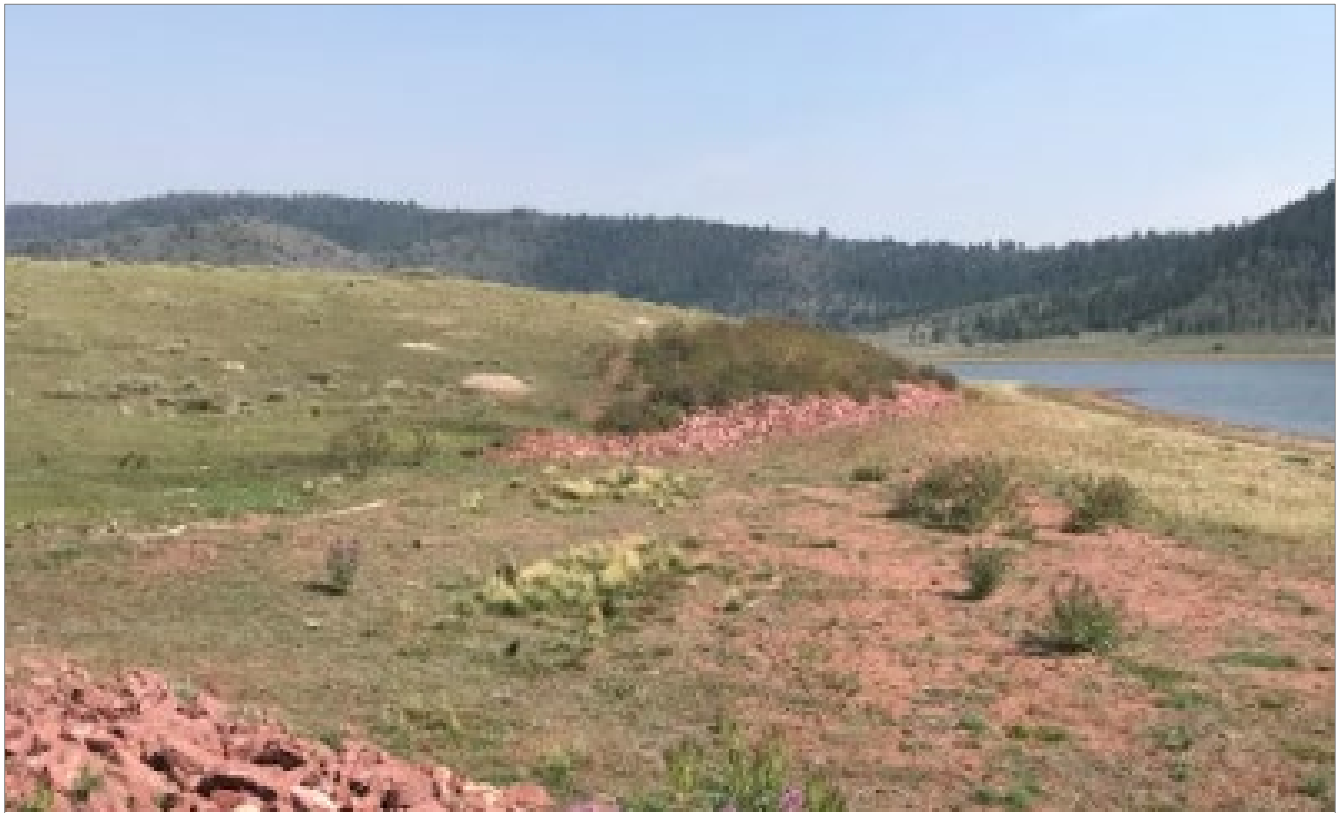
Northern shoreline following recontouring, riprapping, and reseeding.
