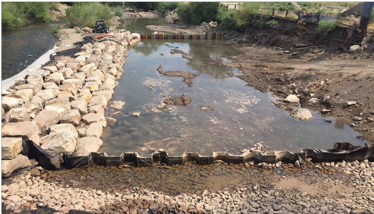
Construction on the three levels of the Kayak Park
