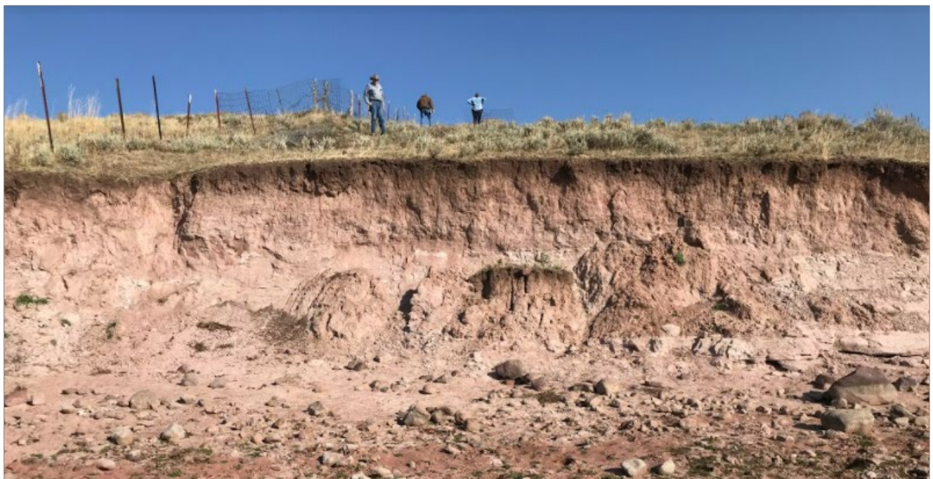
Northern shoreline prior to bank stabilization
