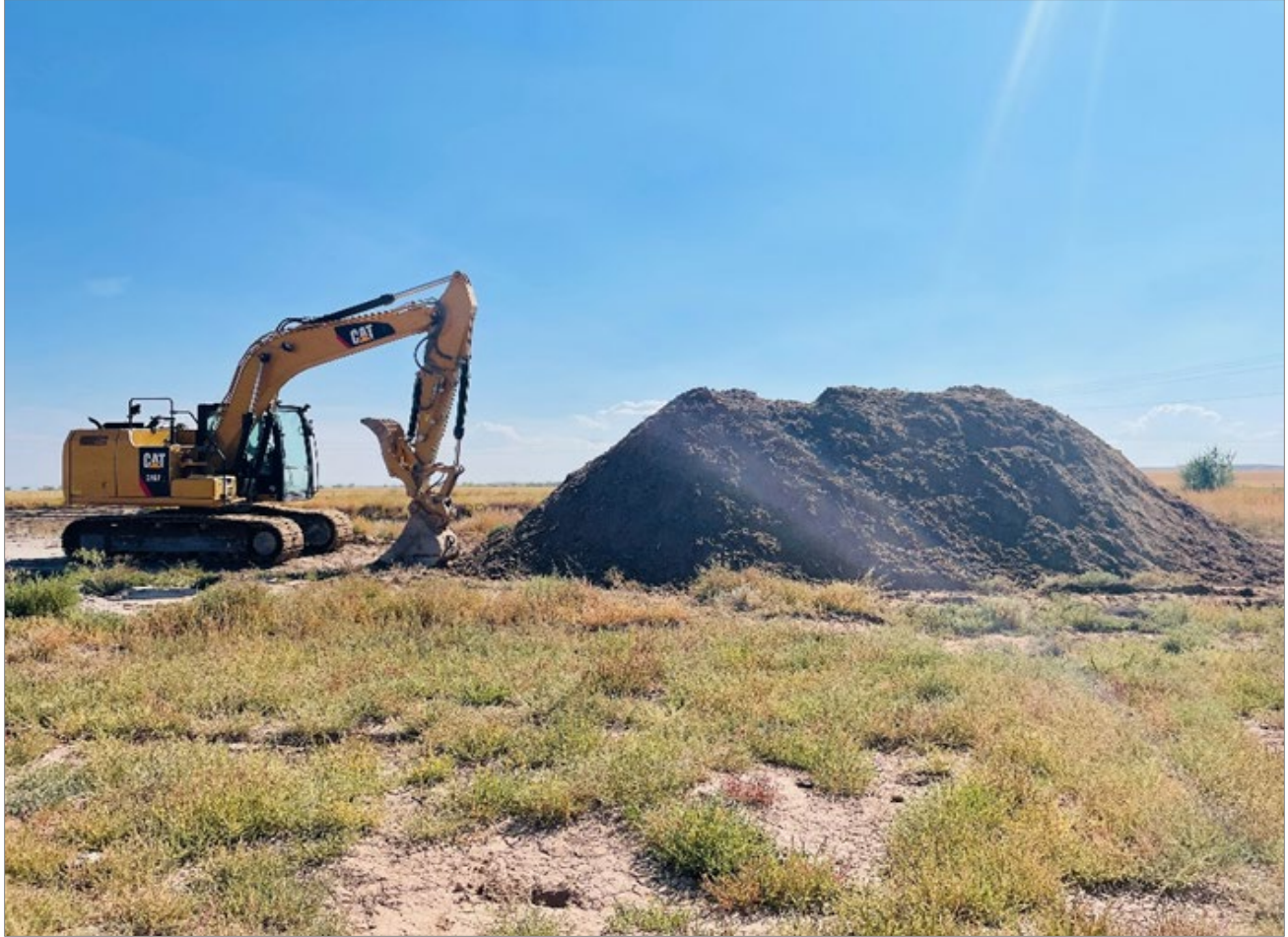
Total amount of heavy sands excavated from the Pelican Lake sediment catch basin in 2021
