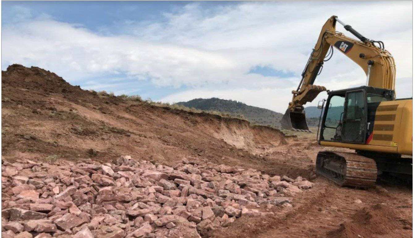
Heavy equipment positioned bedrock riprap and recontoured the shoreline.
