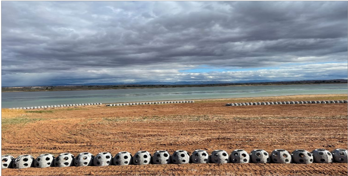
Reef ball structures at three in-lake elevations and one high-water shoreline elevation.
